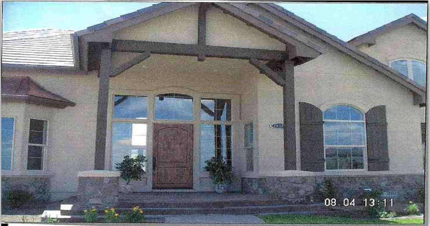
VIEW OF FRONT ENTRY
